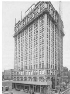
Figura 2: Southwestern Bell Telephone Company 1928, Kansas City USA.
