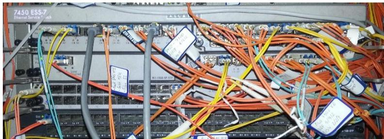
**Figura 77:** Switch Alcatel-Lucent 7450 ESS-7.
