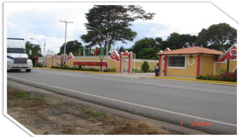
Figura 4. Fachada del Hotel Marivir Suites
