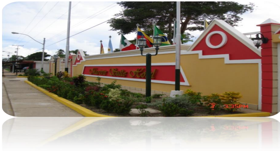
Figura 3. Fachada del Hotel Marivir Suites
